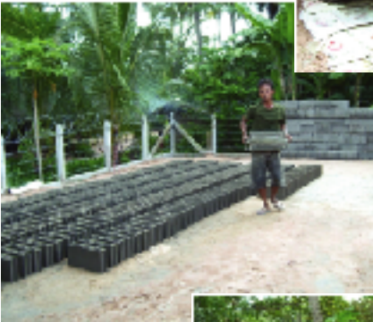
These concrete blocks are stacked and ready for wall construction.
