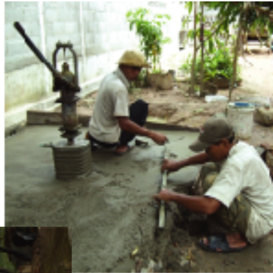
A manual water pump is necessary to maintain a constant water supply during any power outage.
